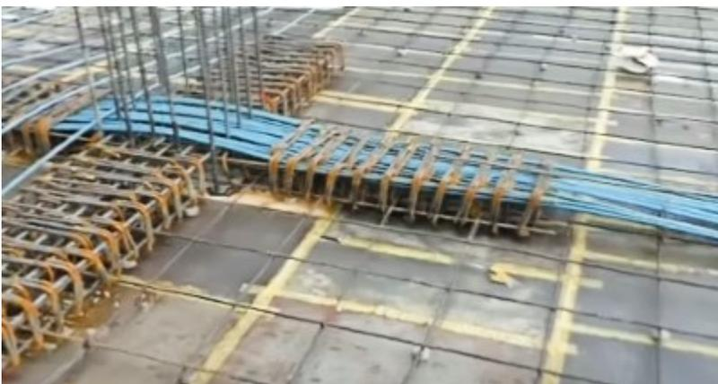
But nowadays slabs are provided tension with the help of tendons to reduce the amount of tension providing materials like steel rods.
